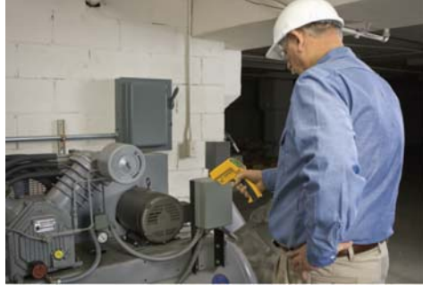
Checking motor temperature.
