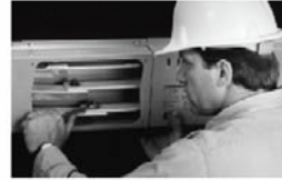
Busway sections bolted together
